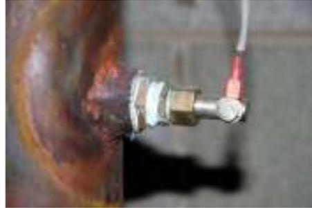
When servicing main domestic line for the entire building, install as close to the water meter or entrance into the building as possible. Liqui-Matic only services what goes through and is beyond the unit installation. The unit has a schedule 80 plastic separator for the probe. The unit must be grounded, but the probe must be separated. (DO NOT replace plastic separator with metal bushing. This will weaken the efficiency of the probe and product).
