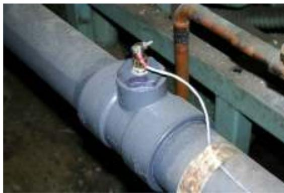
Shut off the water to the area of the application. Install the probe. Attach the box on the wall near the
